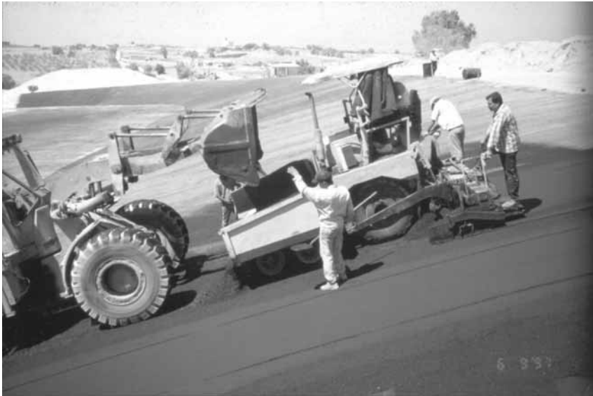
Photo 3.6 Asphalt liners for a sanitary landfill
