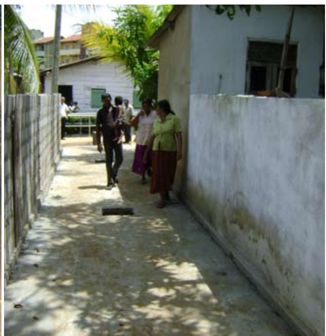
After upgrading through community contracting. Photo © UN-HABITAT/ Lunawa Project
