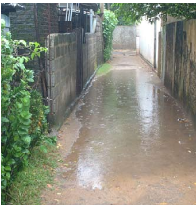
Flooded settlement before upgrading. Photo © UN-HABITAT/ Lunawa Project
